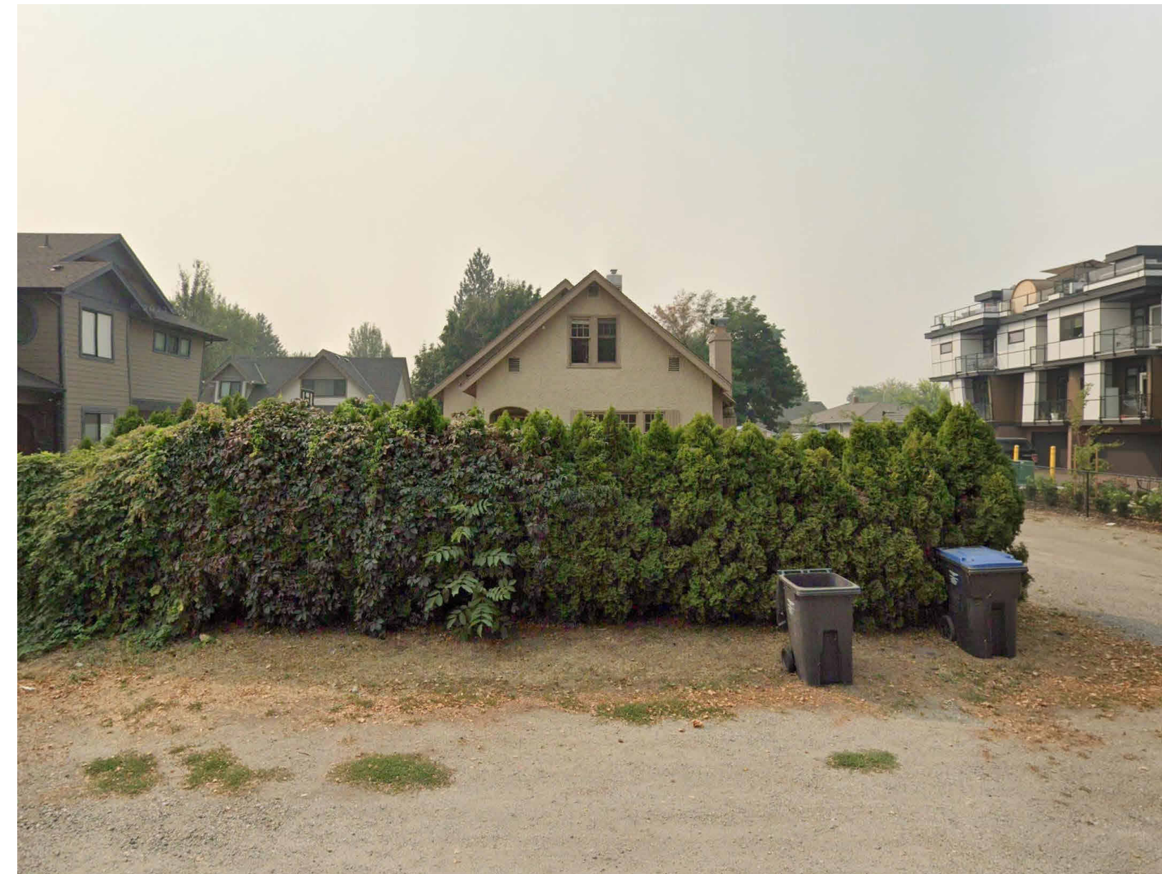
2. VIEW FROM LAURIER AVE FACING THE SITE
