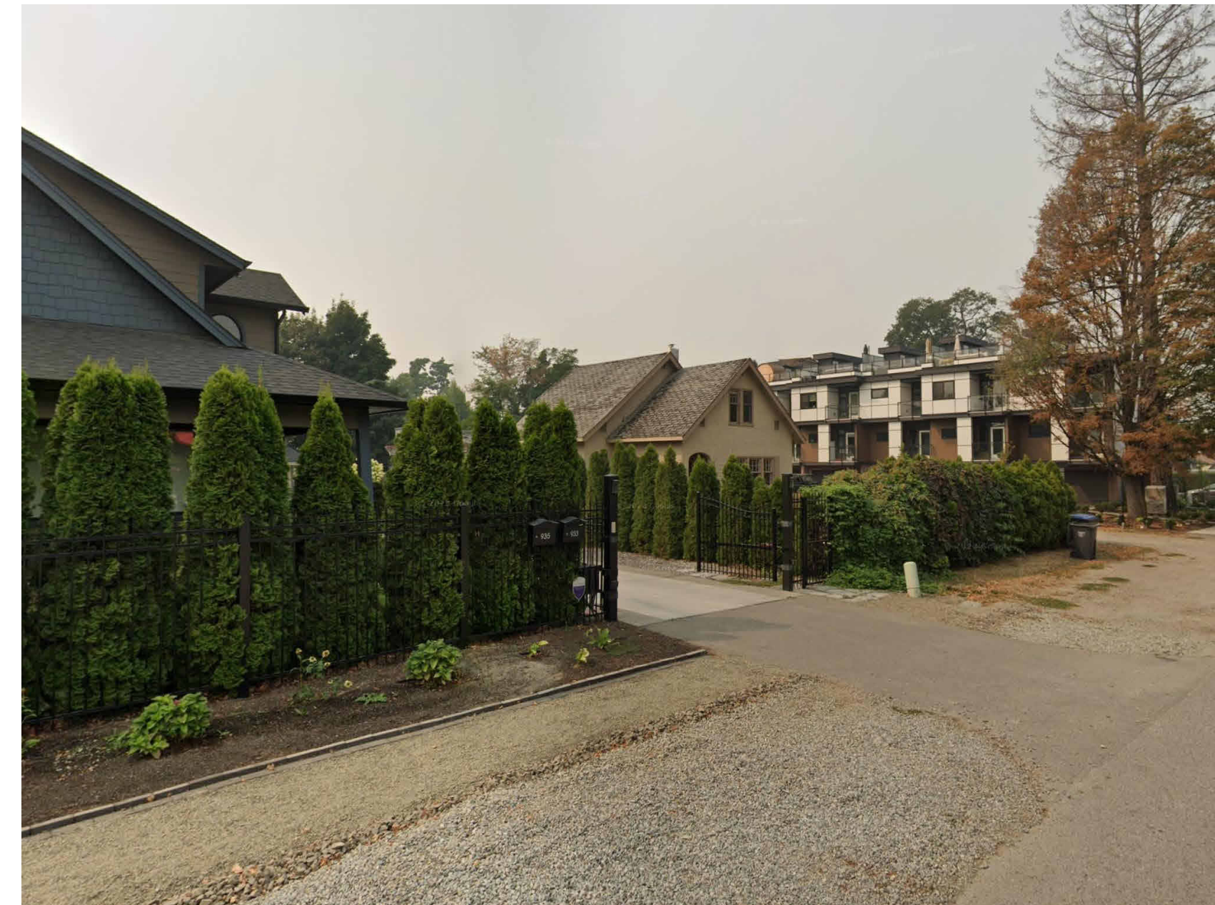
1. VIEW FROM LAURIER AVE FACING THE SITE
